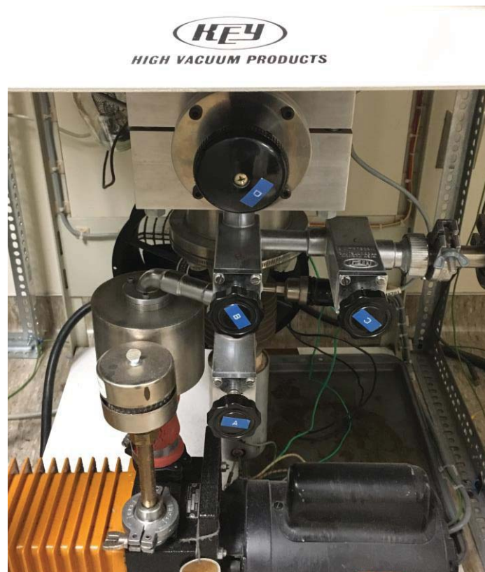
FIG. A.9. Pump system valves (center), mechanical pump, bottom.
