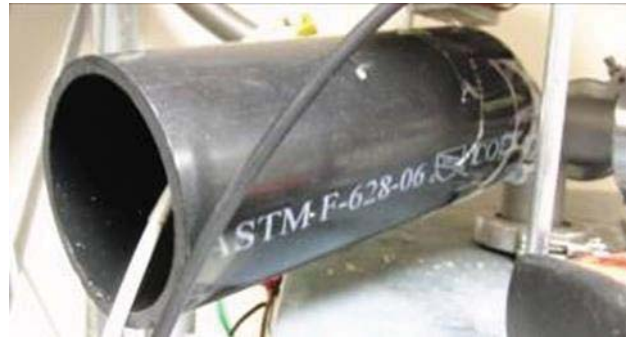
FIG. A.21. High voltage feed through PVC safety cover.
